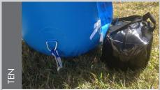
As soon as pressure is correct proceed to attach sandbags or pins to legs using D Rings.
