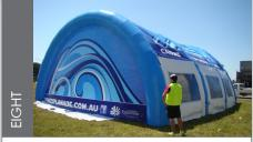
Ensure all legs are lined up and roof is centred. Check frame is firm (do not overinflate).
