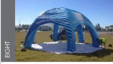
Ensure all legs are lined up and roof is centred. Check frame is firm (do not overinflate).
