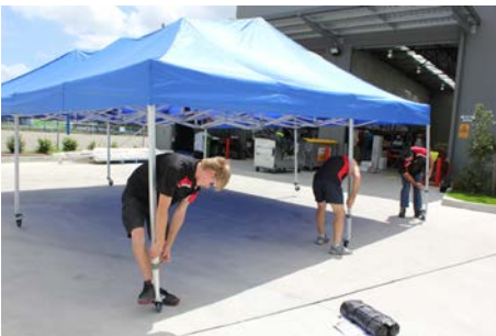
9. Extend the front legs halfway. Repeat for back and middle legs. Using one foot, stand on the marquee foot plate, release the pull ring on the middle leg connector and extend front legs to desired height.
