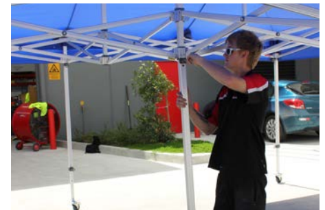
11. Insert the centre leg and extend completely. REFER TO SECURING YOUR MARQUEE ON PAGE 1.
