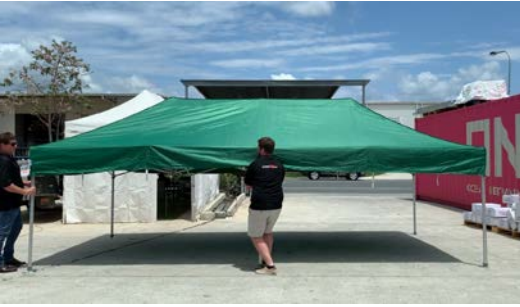
9. Middle Legs. Lift the front back roof connectors until pin locks in to position.
