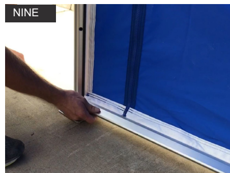
NINE Bottom of Full Wall. Insert the Full Wall Keda into the Support Bar and slide Bar along fabric.
