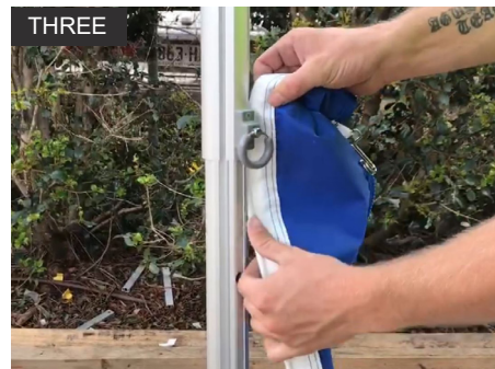
THREE Insert the top of the Wall Strip Keda into the tracking of the Upper Leg of Marquee. (Hook facing inwards)
