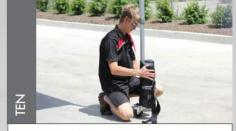
Fit Tie Down Straps, Sandbags, Steel Pins or Weight Plates and anchor marquee into position.
