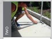
Insert the steel lock bar into the lock connector. Repeat on all four sides.
