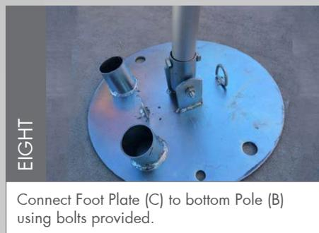
Connect Foot Plate (C) to bottom Pole (B) using bolts provided.
