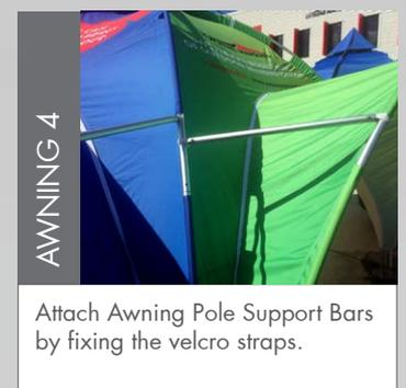
Attach Awning Pole Support Bars by fixing the velcro straps.
